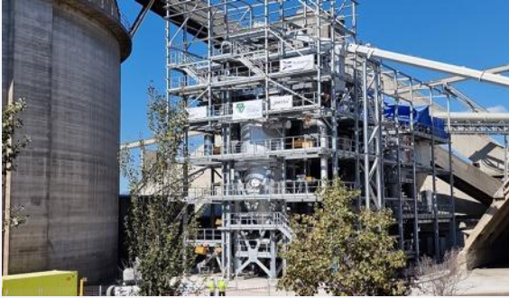
SRF Gasifier Plant 30 MWth SYNGAS to Cement kiln. Spain. Startup March 2026
