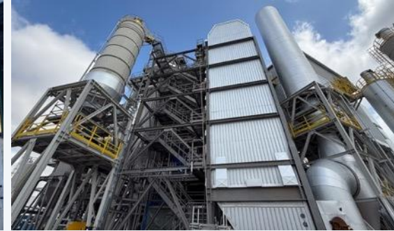
MBM Gasifier Plant 25 MWth Steam + 2MWe. St Langis lès Mortagne France
