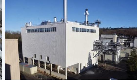
MBM Gasifier Plant 18 MWth Steam + 2 MWe. Lyss, Switzerland
