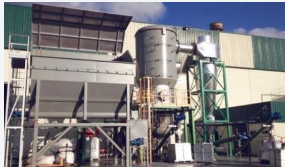
MBM Gasifier Plant 10 MWth Steam. Salamanca, España
